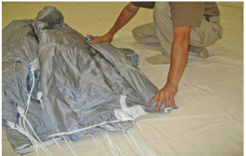
Figure 2-62. Long Fold The A-B Fabric Fold
